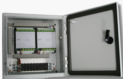
Additional steel wall casing, open
