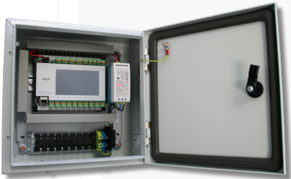
Steel wall casing, open
