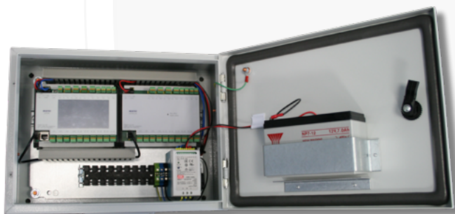
Steel wall casing, open
